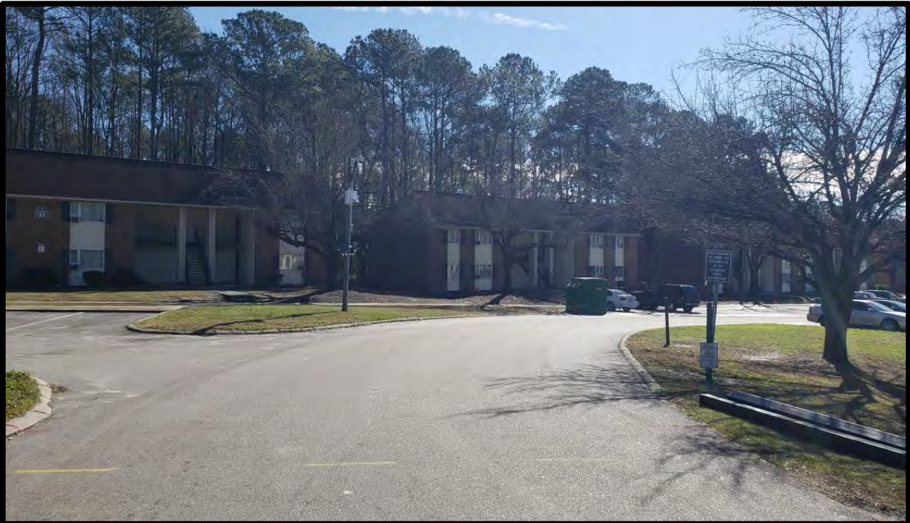
Photo 14 – the subject entrance from Lester Drive
