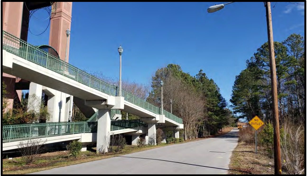
Photo 15 – looking north on Lester Drive with pedestrian bridge across highway on the left
