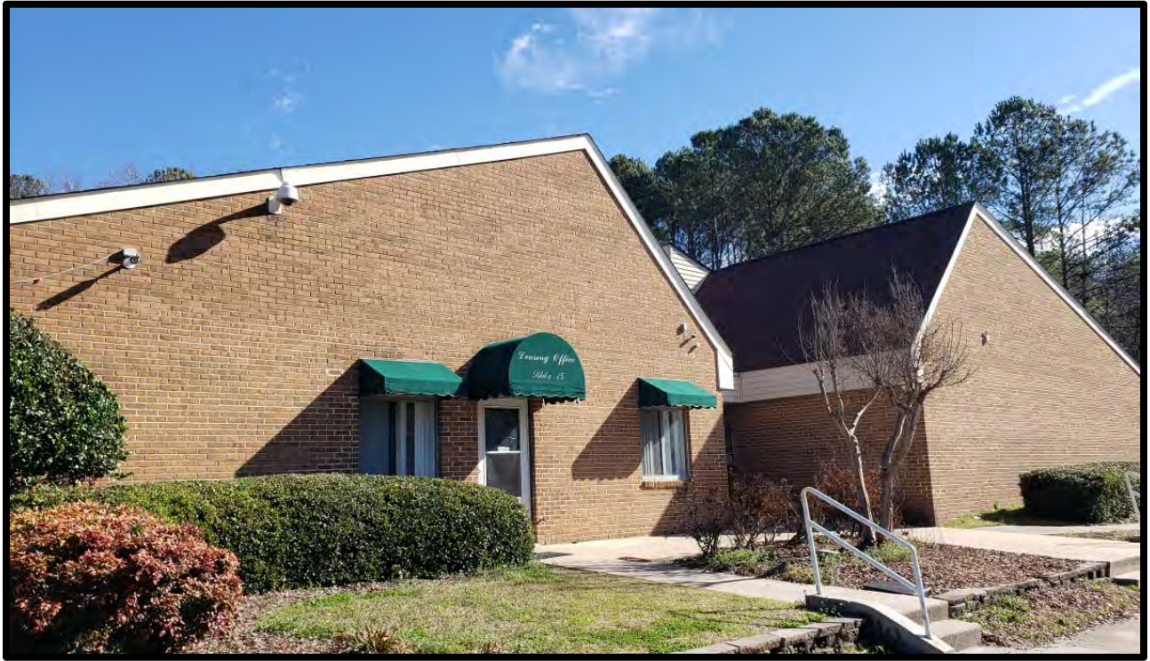
Photo 1 – the subject’s leasing office
